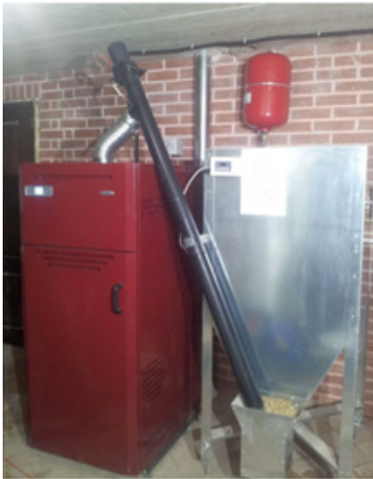
Figure 15. On the top, an adjoining 130 kg tank (Source: Arc Habitat). On the bottom, an additional 300 kg silo with worm auger feeding (+ 2000€ HT).
