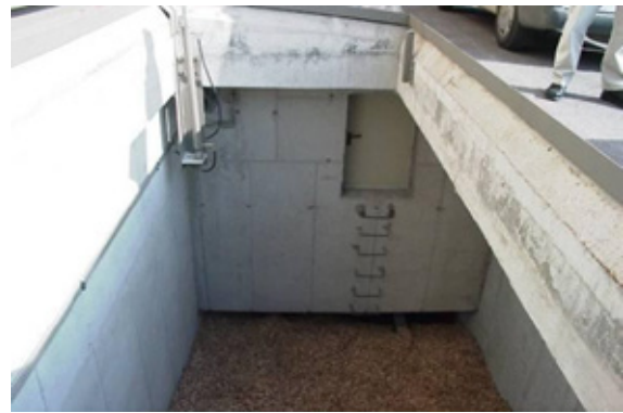
Figure 18. Silo with crossbow system to allow good feeding of boiler
