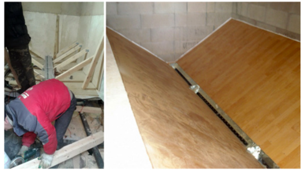
Figure 20. Installation of an adjoining room with a funnel and screw system
