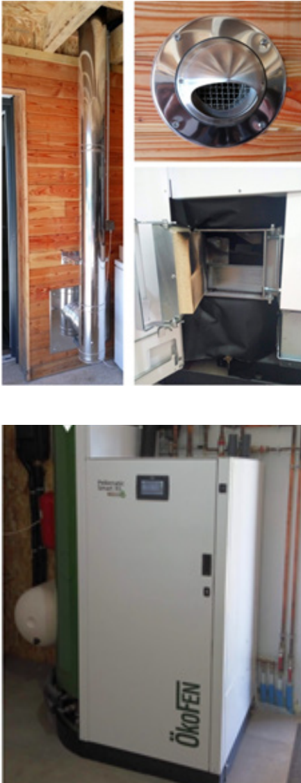
Figure 25. ÖkoFEN Smart XS pellet boiler with integrated 335L storage tank
